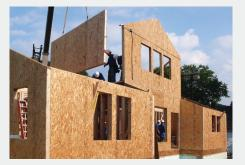
Typical SIP wall TWICE as strong as stickframe stud wall and maintains strength after flooding.
