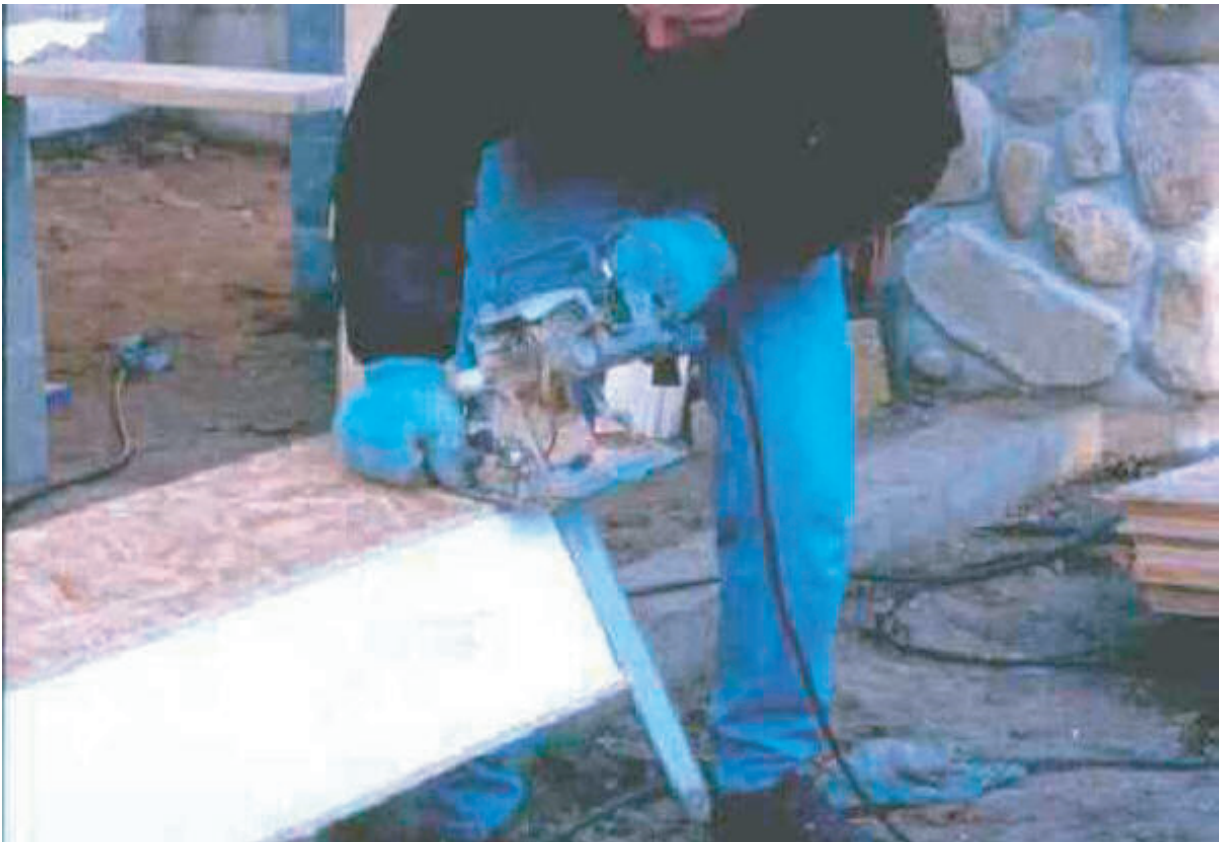
Field cutting SIPs with a modified circular saw
