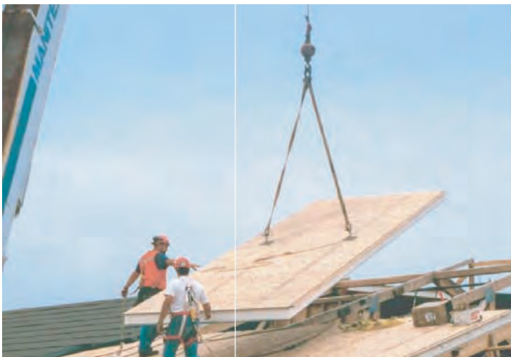
Lifting a SIP with Lifting Plates
