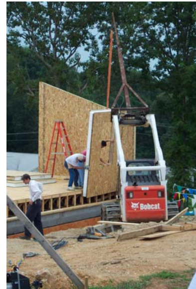
Figure 42. Mounting the wall panels on the side of the floor trusses leaves easy access to run electric wires from the walkout lower level into the vertical wiring chases in the wall SIPs.
