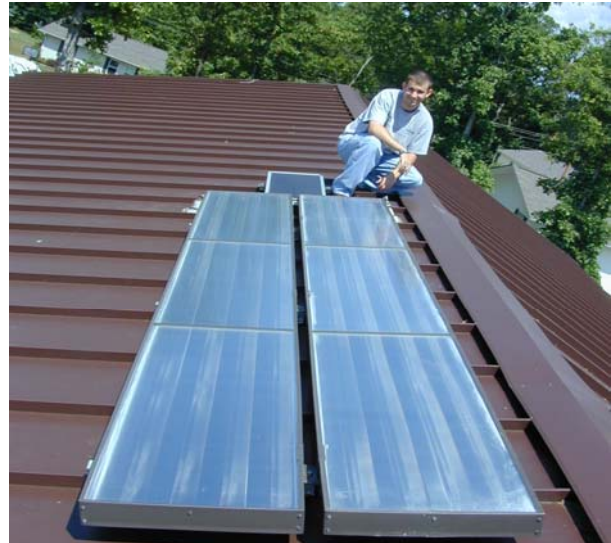
Figure 49. SolarRoofs, SkyLine System 5 solar water heater, with 38 ft 2 of solar collector area installed on the roof of ZEH5.
