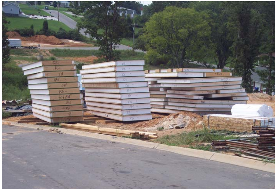
Figure 4. SIP panels for ZEH5 come numbered to match the panel cut drawings. SIPs should be stacked in the order in which they will be installed.
