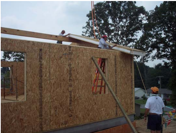
Figure 32. The SIP roof panel installation.
