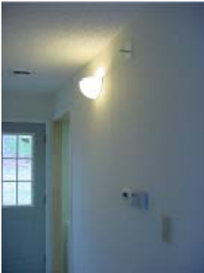
Figure 43. Sconces with compact fluorescents.
