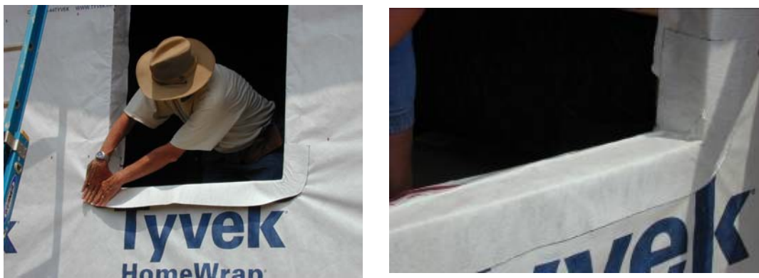
Figure 28. Panned window opening.
