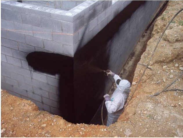
Figure 21. Waterproofing. Note to be OSHA compliant the over cut of the house needs to be sloped 45° for depths greater than 5 ft deep.
